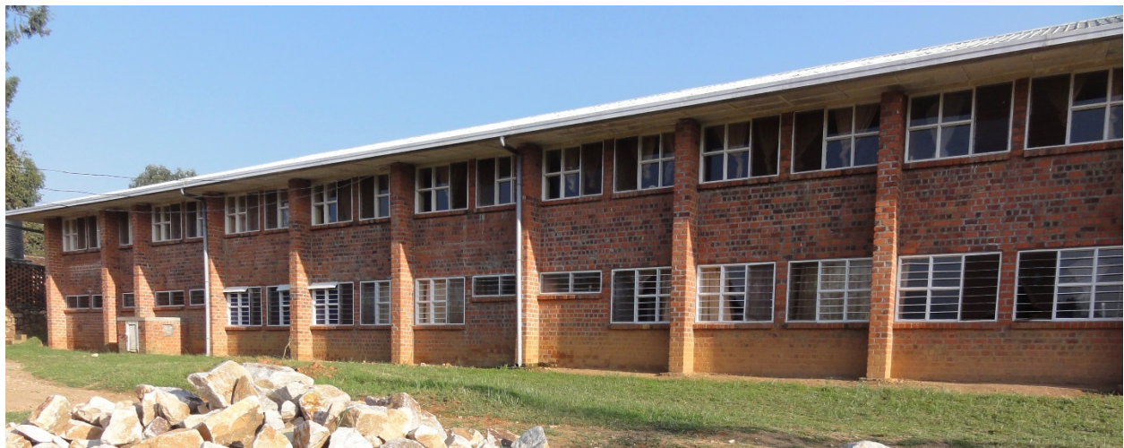
View of the building which will be repurposed to house the new maternity ward
